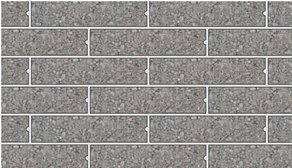
Appearance of PLASCON separating wall as built
